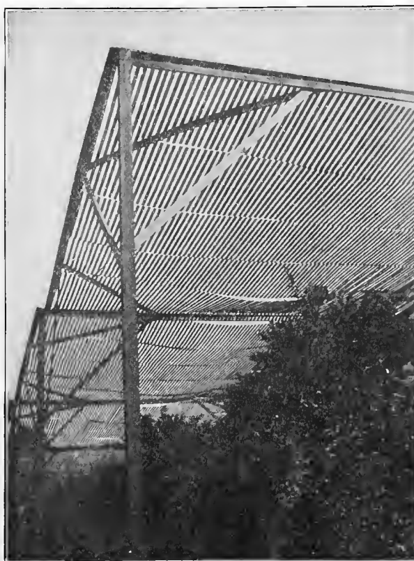
FIG. 19.—Lath screen at ranch of Mr. A. J. Everest, Riverside, Cal. (under view).
